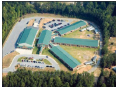
Figure 2. Bessie L. Baggett Elementary School [1].
